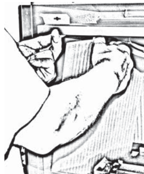
Rotate anchor up and insert panel
