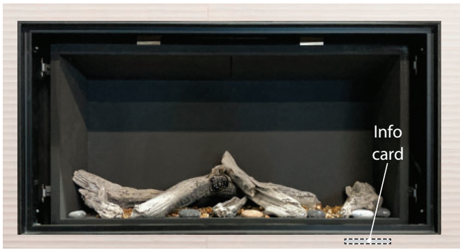
The info card is located behind the front panel below the window.
