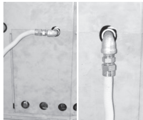
Flex connector redirected using two elbows.
