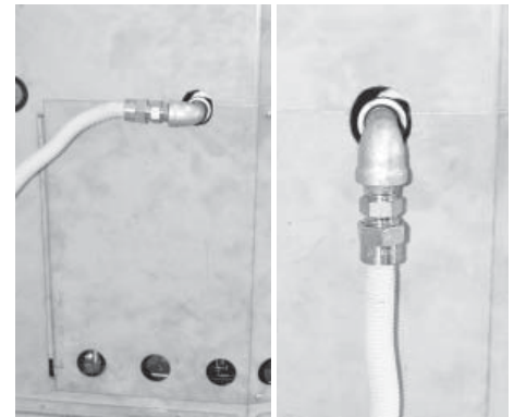
Flex connector redirected using two elbows.
