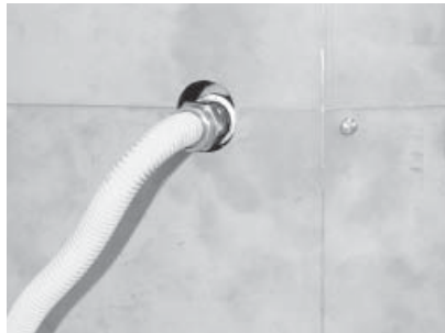
Flex connector redirected using one elbow.
