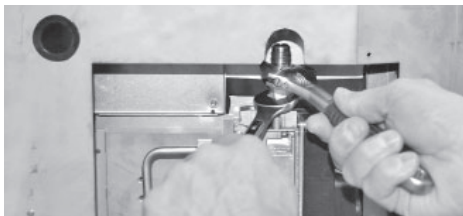
Flex connector redirected using one elbow.
